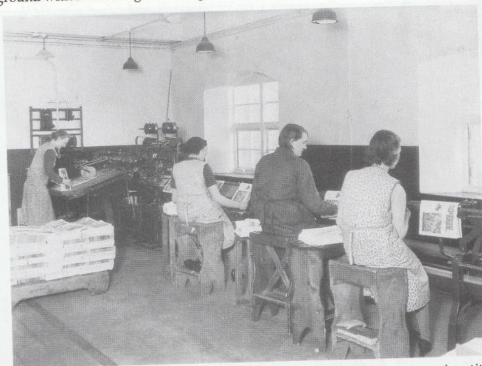
Operating the feeder-stitcher machines, c1938. The sheets and covers were wire stitched at a rate in excess of 3000 complete magazines per hour. Left to right: Edna Hartley, Dot Brown, Gladys Johnson, —.
