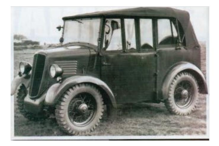
Above: the Morris Wasp was unusual in being a purpose-designed light military staff car. Two prototypes were constructed during 1937, one with a closed saloon body, the other (shown here) equipped as an open-topped tourer. Sadly, there was no series production. These vehicles featured four wheel drive with an auxiliary gearbox and the 8 hp engine.
