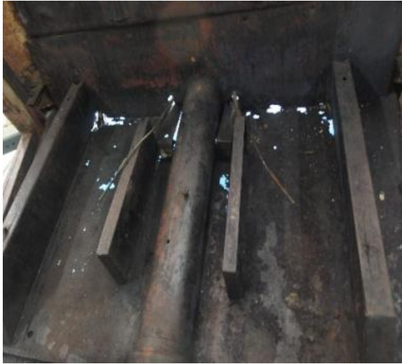
2) Floor: Extensive rust holes apparent.
