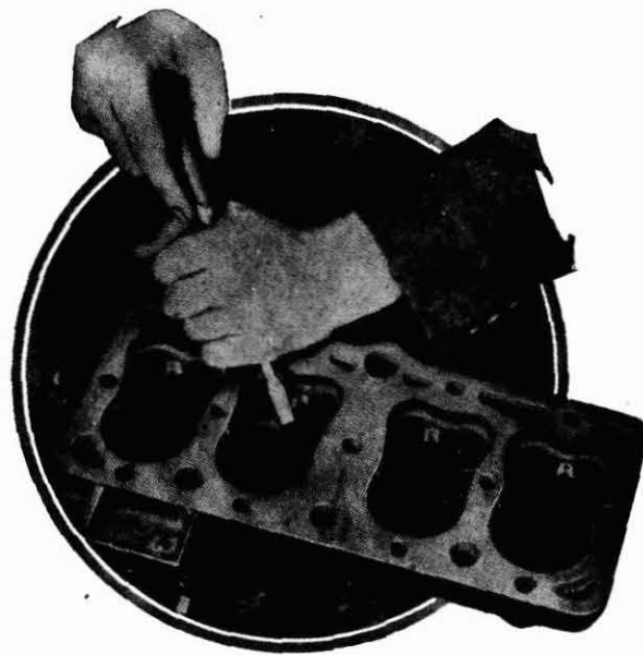
Decarbonising the cylinder head.
